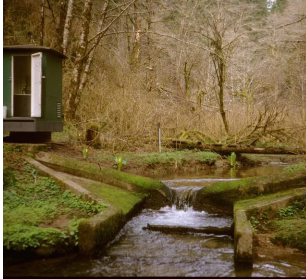
The broad-crested compound weir at Flynn Creek. Note outside staff gauge in the pool on river right.
